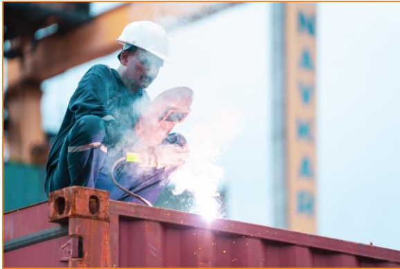
Container's repair and maintenance
