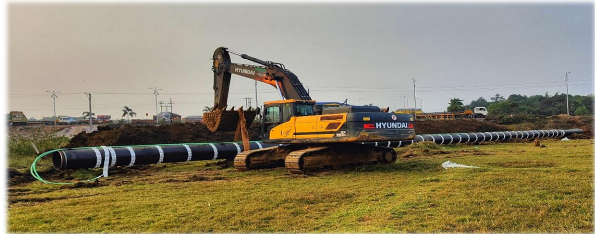
Setting up slurry pipeline
