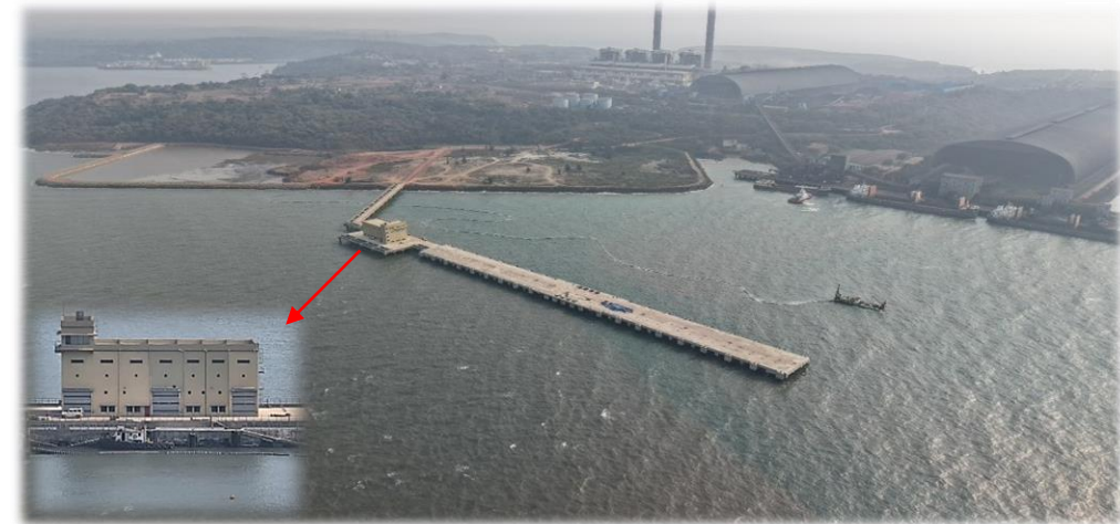
Berth and Pump house at Jaigarh
