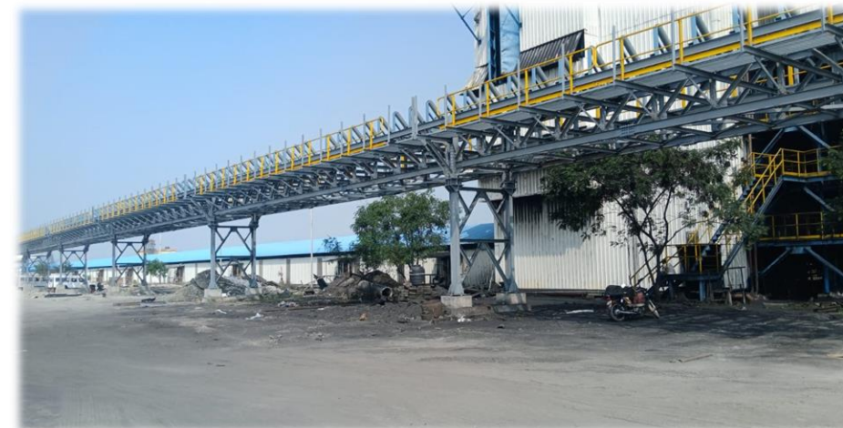
Works under progress at Tuticorin site
