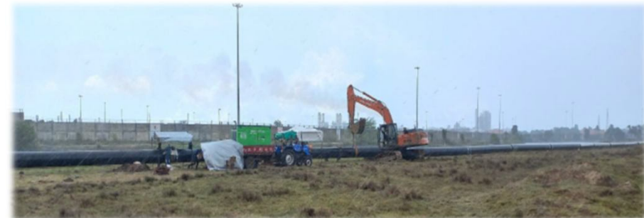
Setting up slurry pipeline
